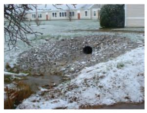
An apron protects and stabilizes the culvert outlet the full width of the bottom and one foot above the maximum outflow elevation.
