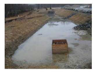
An emergency spillway is necessary unless a piped outlet can pass all peak flows without overtopping the embankment.
