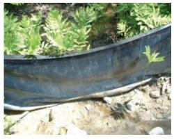
Silt fence can be difficult to install properly in shallow-to-ledge, stony, or forested soils as well as frozen ground. The added disturbance near a water resource is not recommended.
