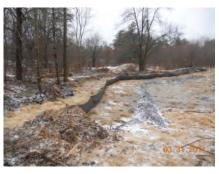
Sediment barriers should be inspected and repaired before, during, and after each rain event.
