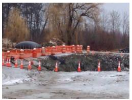
During dewatering, frequently inspect the receiving area for signs of erosion, concentrated flows or sediment discharge and repair immediately.
