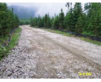
Good road surface and base material contains gravel, sand, and a few fines. Gravel and sand in the subbase provide strength and drainage.
