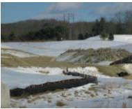
Stabilization during the winter construction period may include mulching, erosion control mix, erosion control blankets, and stone.
