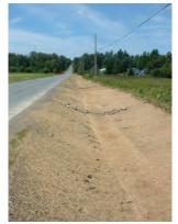
During construction inspect the channel daily and during storm events to check for erosion. Repair as needed. After the channel is stabilized, maintain a channel that is stable and free of debris.
