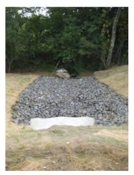
The riprap should extend across the bottom and up both banks of the channel to the maximum height of flow or to a point where vegetation can be established.
