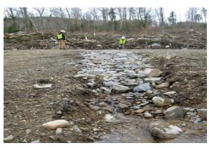
or streams with a large flood plain. A minimum of 6 inches of flow depth over the ford is required for fish passage and should be provided on one side of the ford only. A temporary water ford may be made of timber mats or blasting mats.
