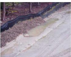
Damaged or otherwise ineffective sediment barriers should be replaced with new material or a different barrier measure.
