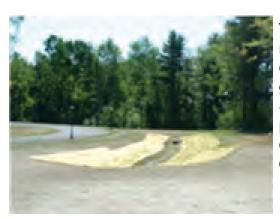
Vegetated swales need to be stabilized early during the growing season (by September 15) or protected with an erosion control blanket or riprap.
