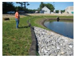
Continuous contained berms may be placed by hand, machinery or the sock may be filled on-site by a pneumatic blower.
