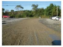
The pad should be inspected weekly as well as before and after a storm. The pad may have to be replaced if the voids become filled with sediment. Street sweeping may be necessary. Site
