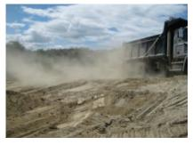
**Stabilize** all laydown areas and all unpaved surfaces with a base gravel or coarse gravel as soon as possible. Use traffic control to restrict speed and route.
