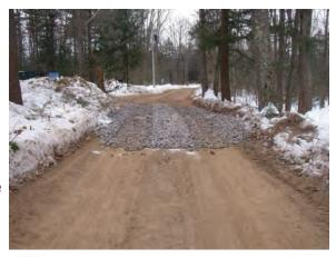
**TEMPORARY FORDS** consist of the reinforcement of the streambed for traffic while maintaining adequate fish passage but should not be used for streams with soft mucky bottom
