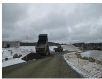
The preferred road construction is above natural ground elevation for positive drainage. Cuts and fills are more of the norm for roads constructed along the contour of sloping sites.
