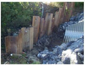
Regularly inspect a sheet piling cofferdam and repair immediately.
