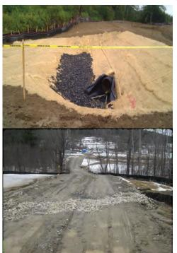
WATERBARS are constructed at a 30-45 degree angle to intercept and direct runoff out of the travel way and for dissipation to the side. Waterbars should be spaced every 250 feet on a 2% road and every 30-40 feet for roads with a 20% grade. In bends or where surface runoff needs shed to one side, the road may be superelevated. Broad-based dips have a wider base than waterbars and are more appropriate on year-round roads.
