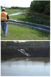
The slope drain should be located on undisturbed soil or wellcompacted fill.
