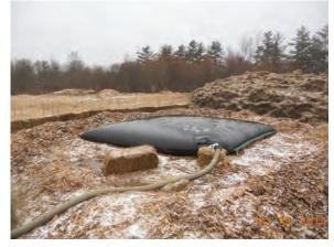
Filter bags have a finite capacity for sediment collection and may be prone to plugging. Avoid over-pressurizing the bag or it may burst. If a sediment discharge is observed, inspect the filter bag for tears or other malfunctions.
