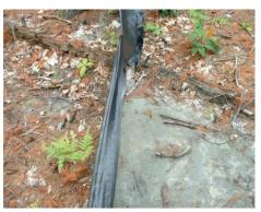
Collected sediments should be removed when one-half the height of the barrier is filled.
