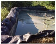
Inspect the structure on a daily basis to assess usage and identify leaks and breaches. Dispose of the solids appropriately.
