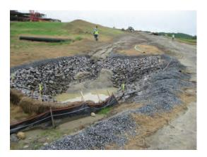
Remove sediments when accumulation reaches the midpoint depth of the trap.
