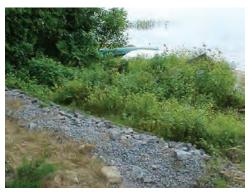
Level spreaders should be constructed on undisturbed soil. The buffer and area below the spreader should remain uncompacted from construction equipment.
