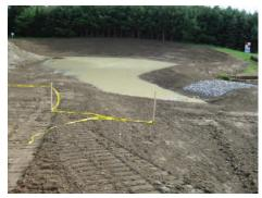
Construct and stabilize a sediment containment structure before disturbing the site and stabilize before a rainfall event.
