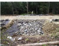
A rock sandwich can provide a permeable road base if built of coarse rocks and wrapped in geotextile fabric to let water drain downgradient.
