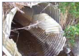
damaged culvert
