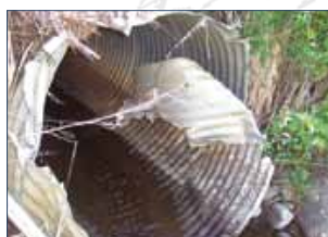
damaged culvert
