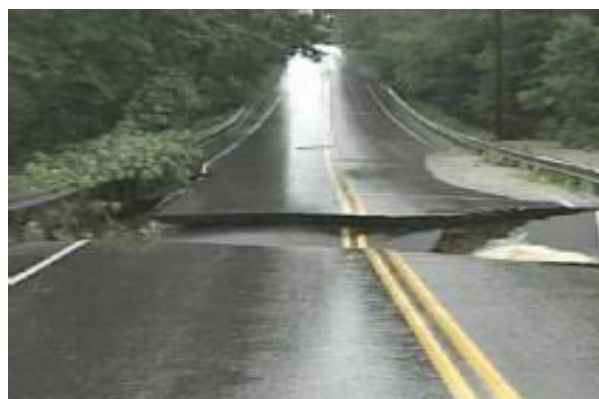
Roads vulnerable to washouts and flooding
