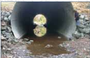
culvert properly embedded into streambed
