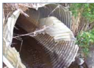
damaged culvert
