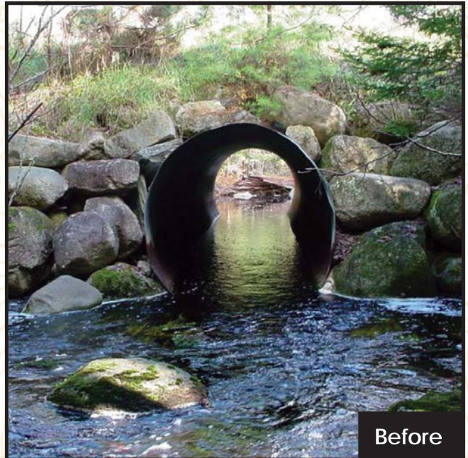
This undersized round culvert prevented Atlantic salmon and native Eastern brook trout from accessing important habitat.
