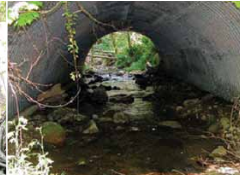
open-arch culvert
