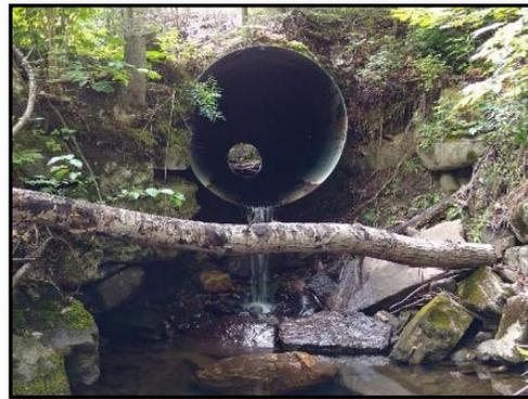
Narrow culverts become perched, preventing passage of fish and wildlife and backing up during high water events.
