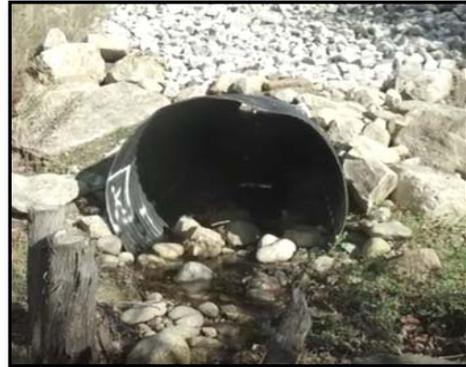
Completed culvert showing streambed material (rocks and sediment) and riprap added.
