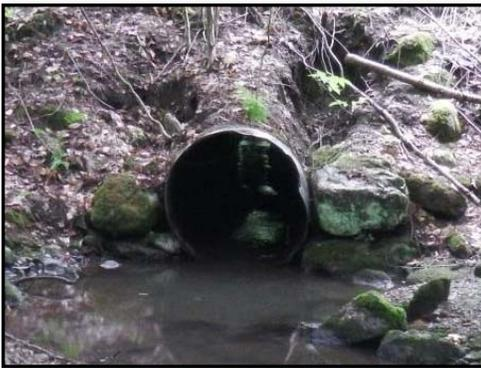
Culvert is too narrow causing pool at inlet. Water backs up during high flow, leading to erosion around culvert and washouts.
