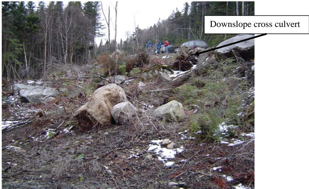
**Photo 6A: Downslope cross culvert with stabilized channel utilizing vegetation. Photograph by Albert Frick, 11/12/2003.**
