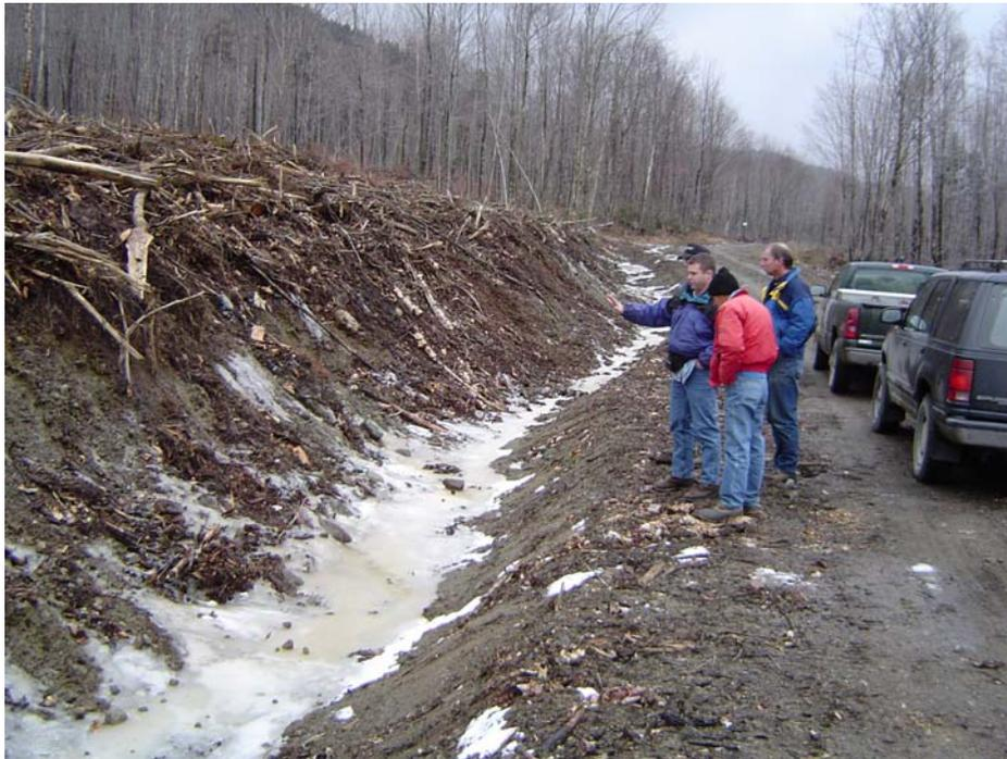
**Photo 7: Recently built existing road cut across moderately well drained soil exhibiting seepage on top of soil underlying glacial till. Erosion and sediment control not yet in place. Photographed by A.F. 11/12/2003.**
