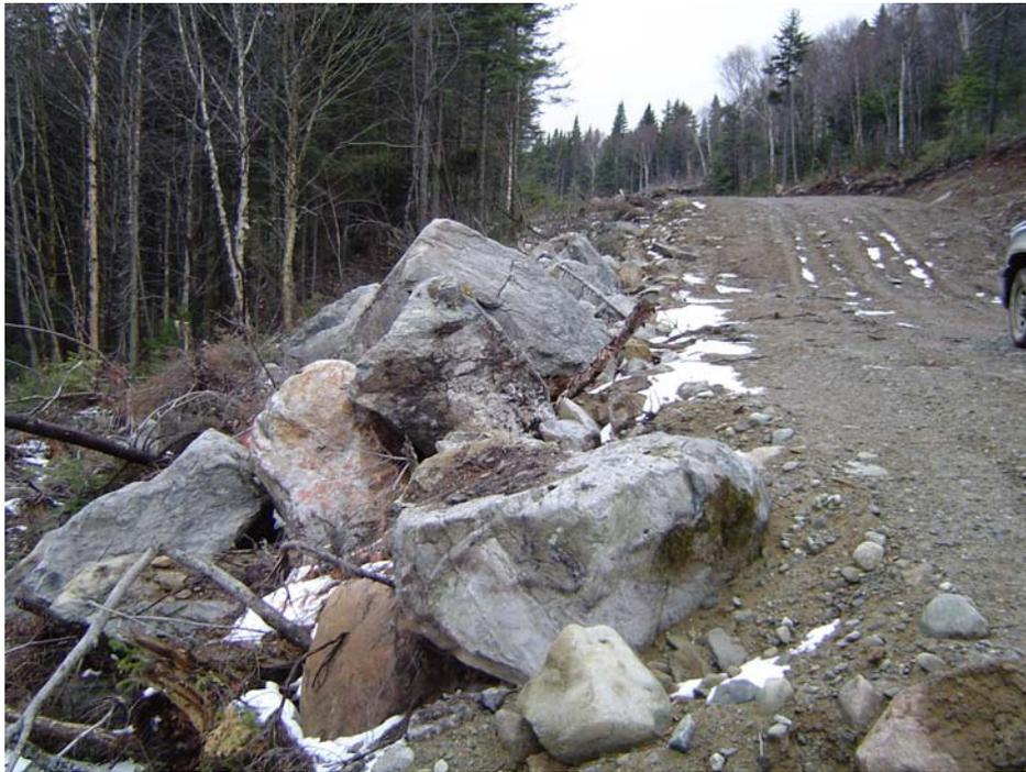
Photo 9: Large boulders utilized on downslope side of fill extension for fill retention and rip rap armament. Photograph by Albert Frick, 11/12/2003.
