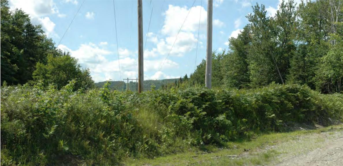
*View of the existing 115 kV transmission line from Rowe Pond Road in Pleasant Ridge Plantation, looking northwest toward Stewart Mountain (to left of clearing in photo). The proposed 115 kV generator lead line will be located within a 100' wide corridor; adjacent to and south of the existing transmission line (on left of corridor in photo).*
