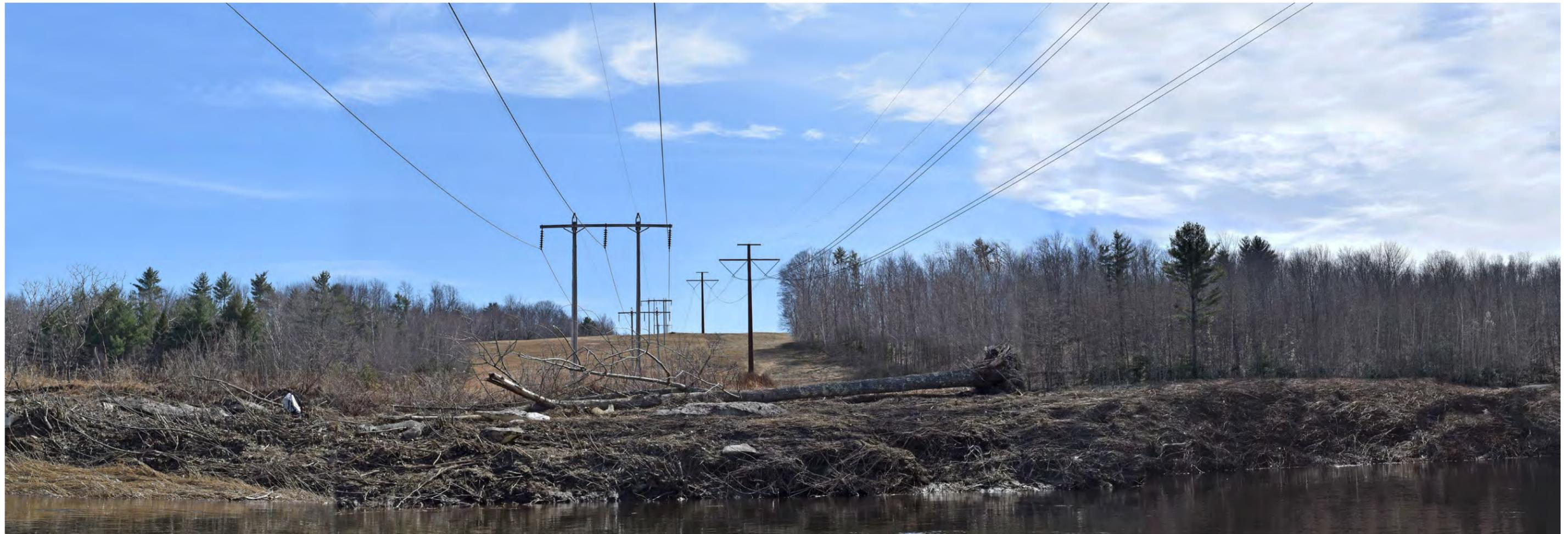
**Proposed Conditions:** Panoramic view looking south to west from the Sandy River in Farmington toward the proposed co-located HVDC transmission line. The existing 225' wide cleared corridor will be widened by 75' on the western side to accommodate the proposed HVDC transmission line. Two proposed HVDC structures and conductors will be visible at distances of 825 to 1,600 feet from this viewpoint.
