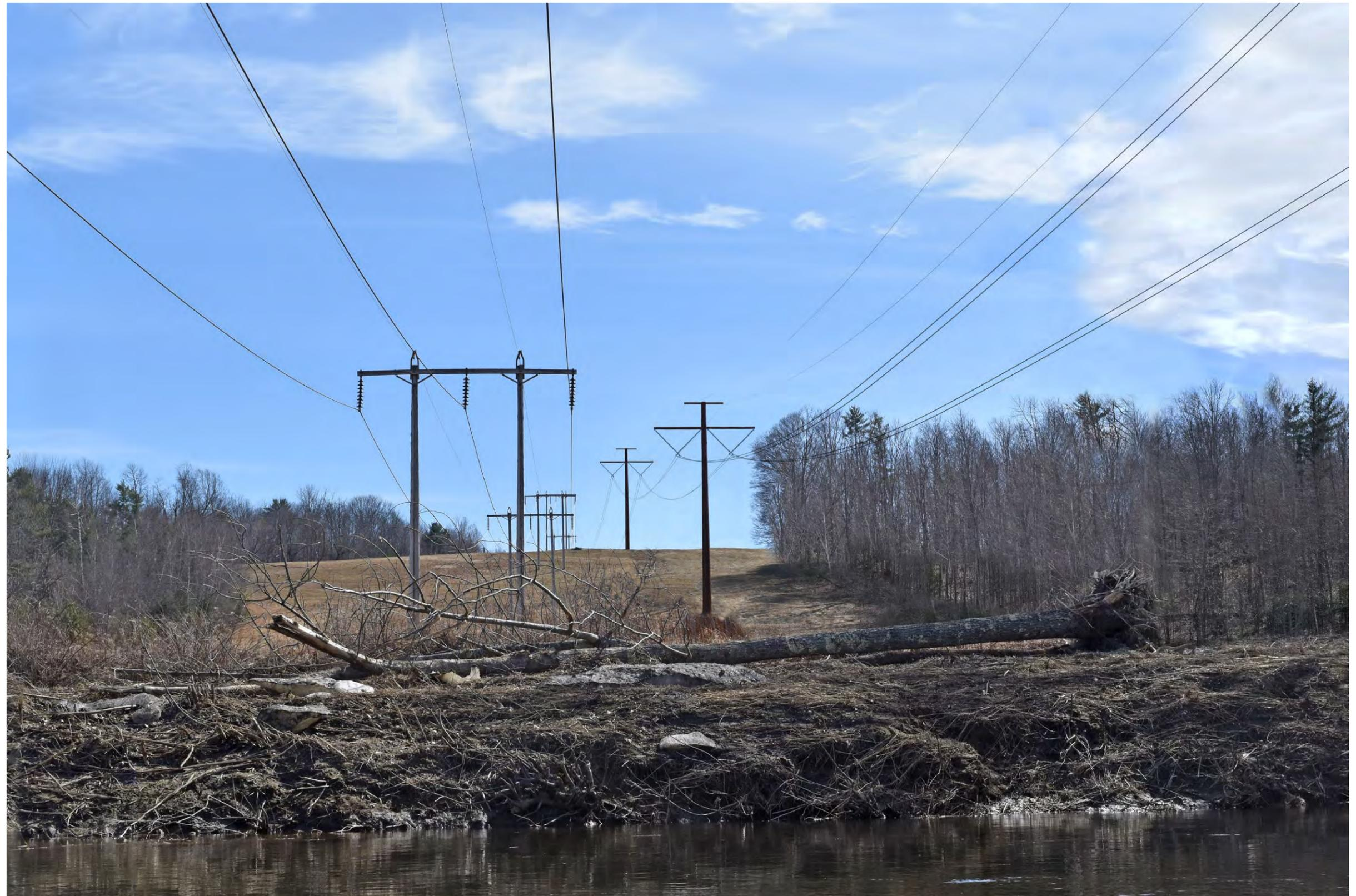
**Proposed Conditions:** Normal view looking south from the Sandy River in Farmington toward the proposed co-located HVDC kV transmission line. The existing 225' wide cleared corridor will be widened by 75' on the western side to accommodate the proposed HVDC transmission line. Two proposed HVDC structures and conductors will be visible at distances of 825 to 1,600 feet away from this viewpoint.
