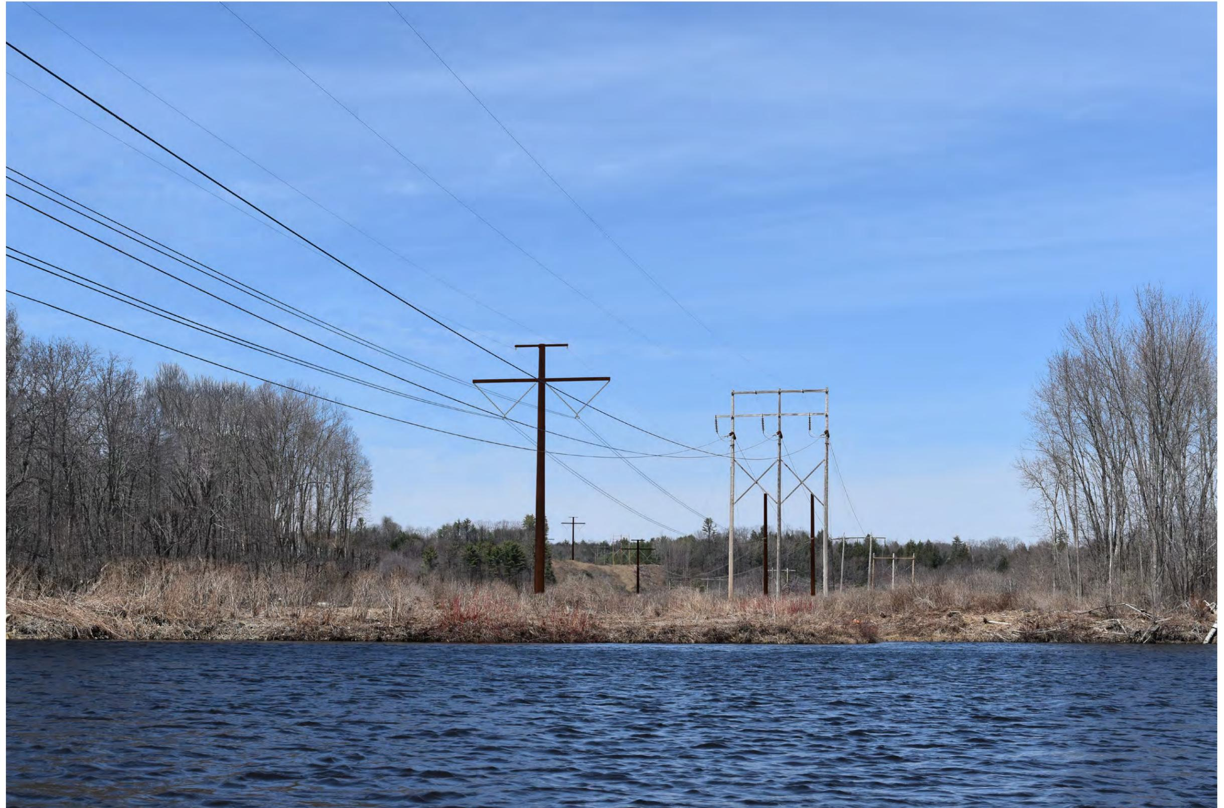
**Proposed Conditions:** Normal view looking north from the Carrabasset River in Anson toward the proposed co-located HVDC transmission line. The existing 225' wide cleared corridor will be widened by 75' on the western side to accommodate the proposed HVDC transmission line. Five proposed HVDC structures and conductors will be visible at distances of 540 feet to 3,160 feet from this viewpoint.
