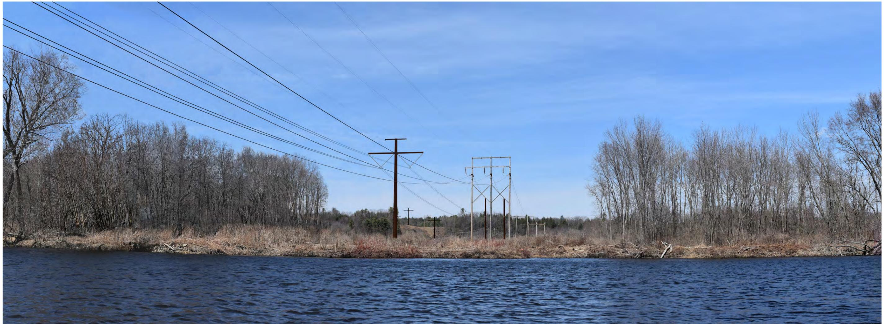
**Proposed Conditions:** Panoramic view looking north to northwest from the Carrabasset River in Anson toward the proposed co-located HVDC transmission line. The existing 225' wide cleared corridor will be widened by 75' on the western side to accommodate the proposed HVDC transmission line. Five proposed HVDC structures and conductors will be visible at distances of 540 feet to 3,160 feet from this viewpoint.
