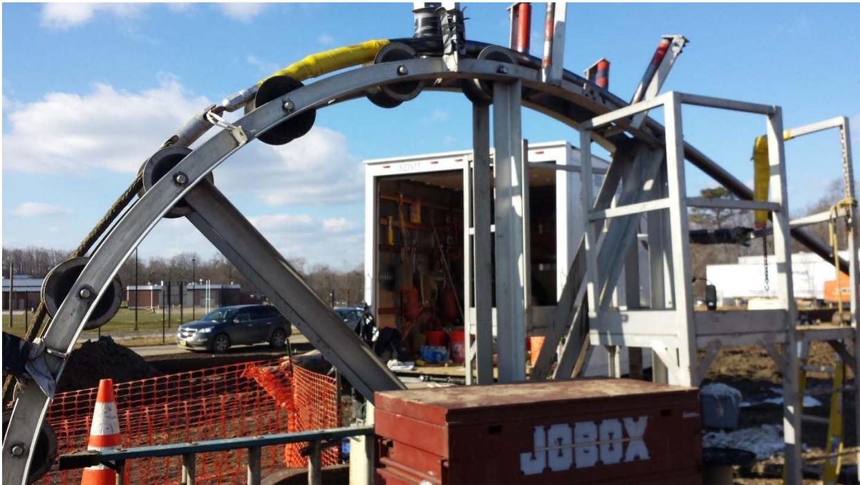
Figure 12- Cable Pulling over Bullwheel
