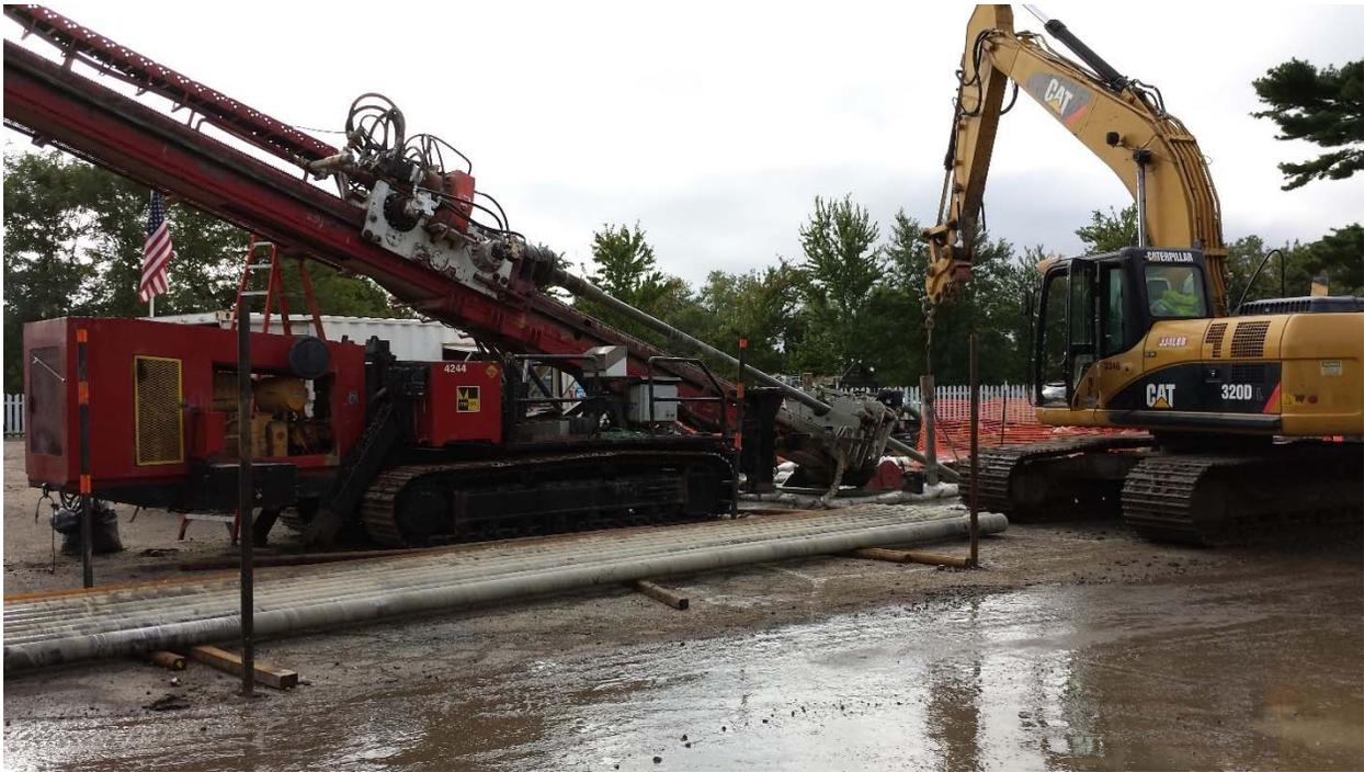
Figure 7 - HDD Drill Rig
