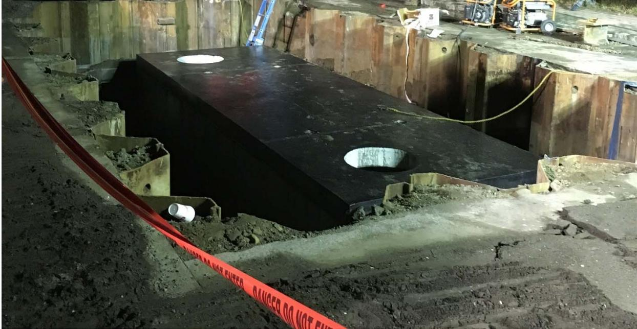
*Figure 5- 115kV Splicing Vault*
