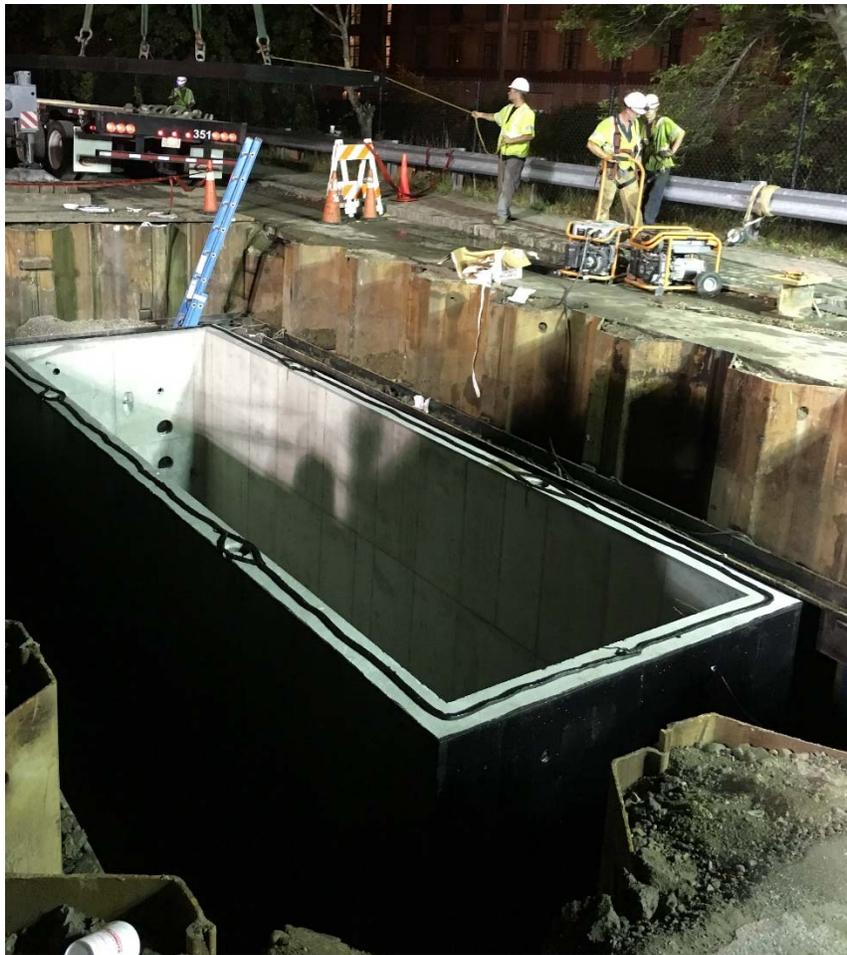
*Figure 4- 115kV Splicing Vault*
