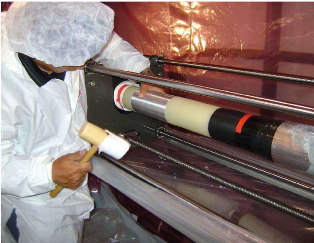
*Figure 14 - Assembling Joint*
