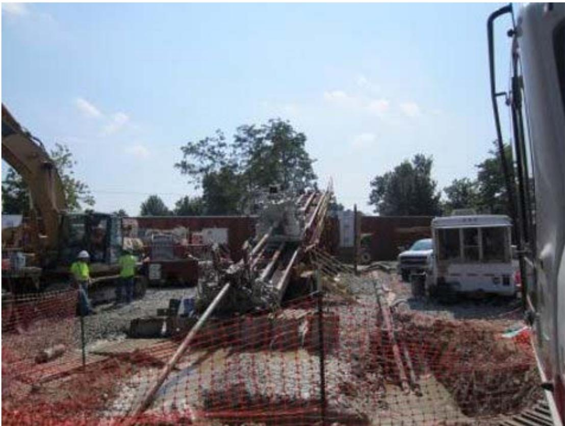
*Figure 6 - Horizontal Directional Drill Rig*
