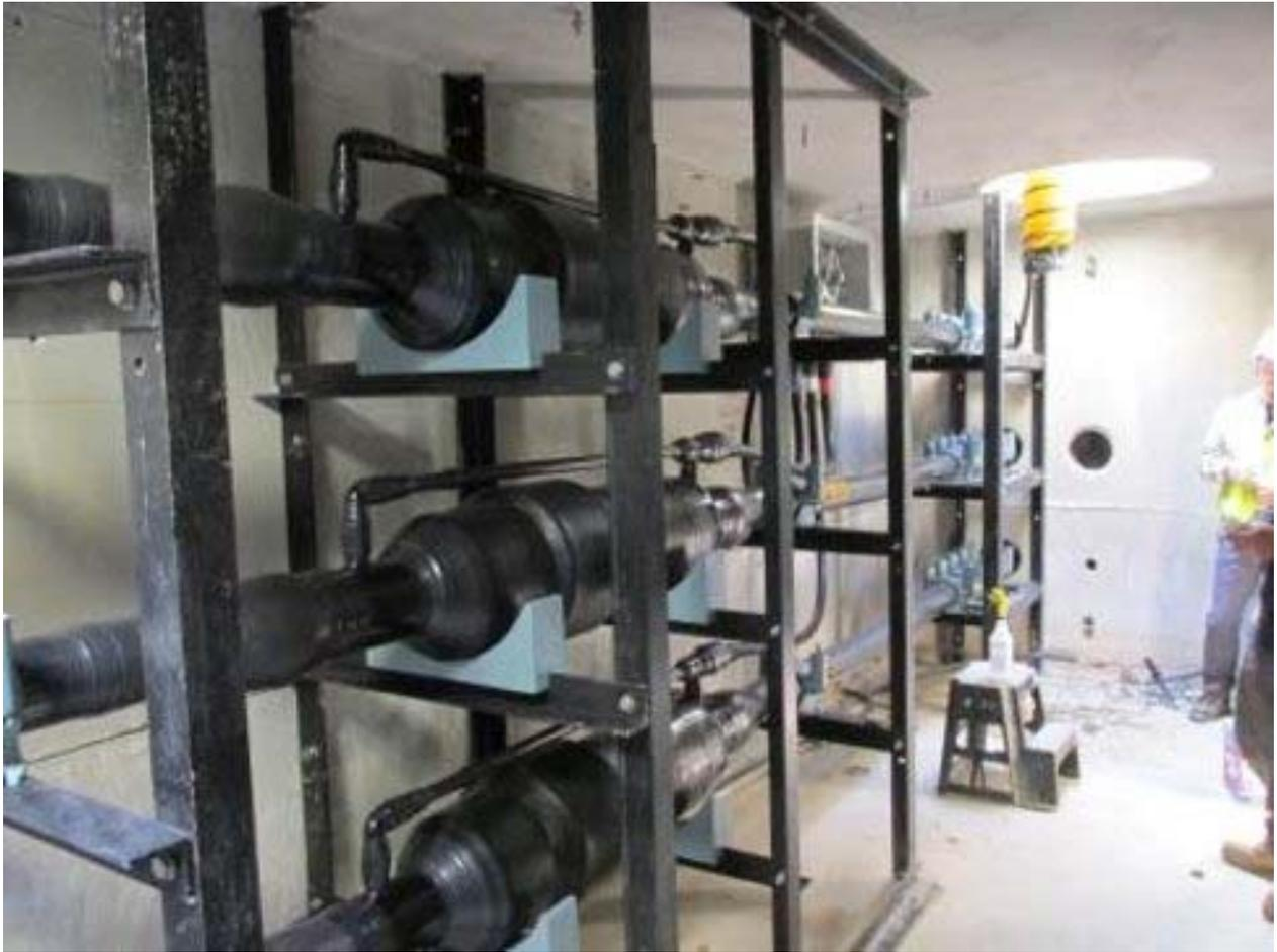
*Figure 15 - Cable Joints in Vault*
