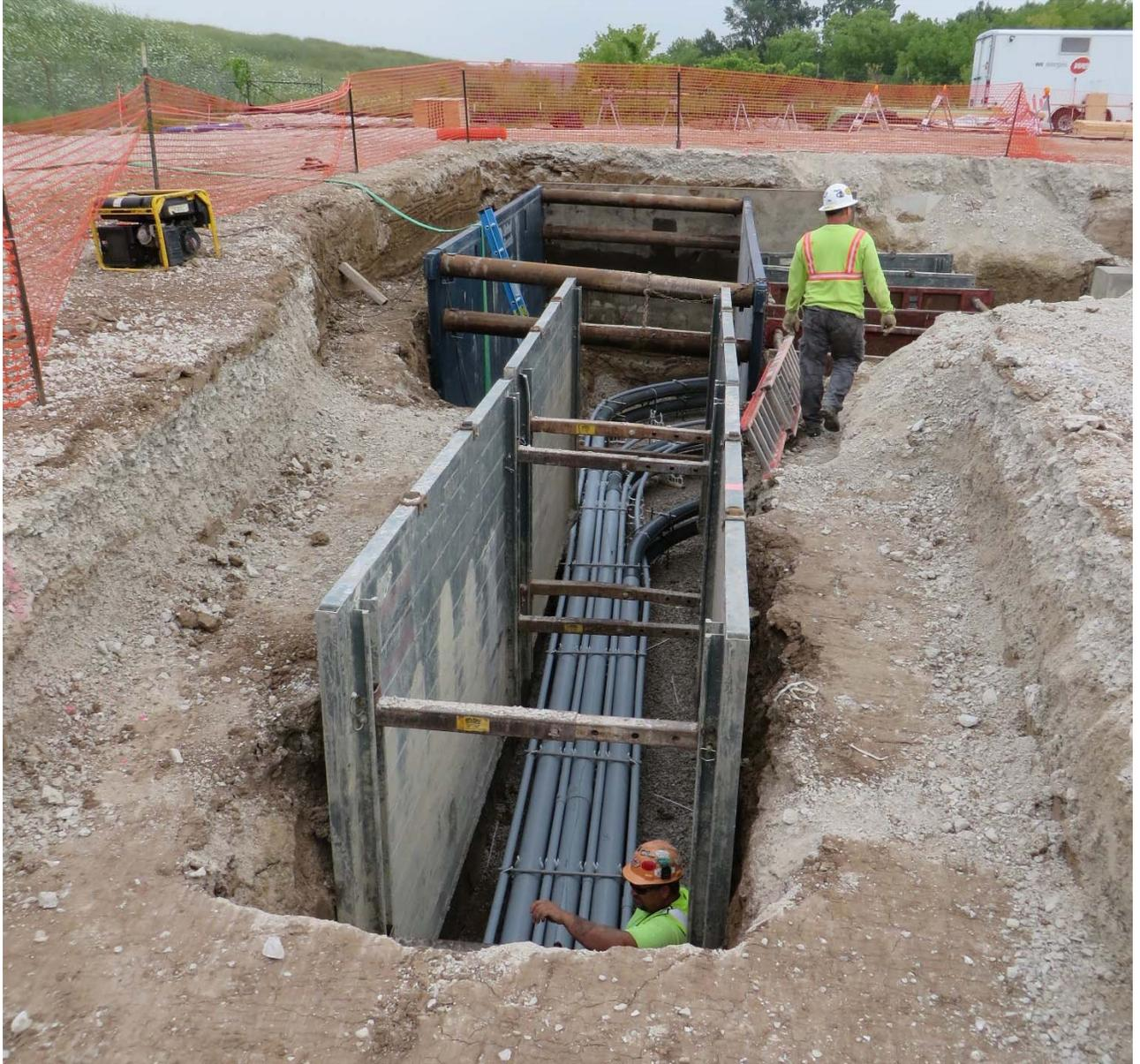
*Figure 2- Duct Bank Excavation*
