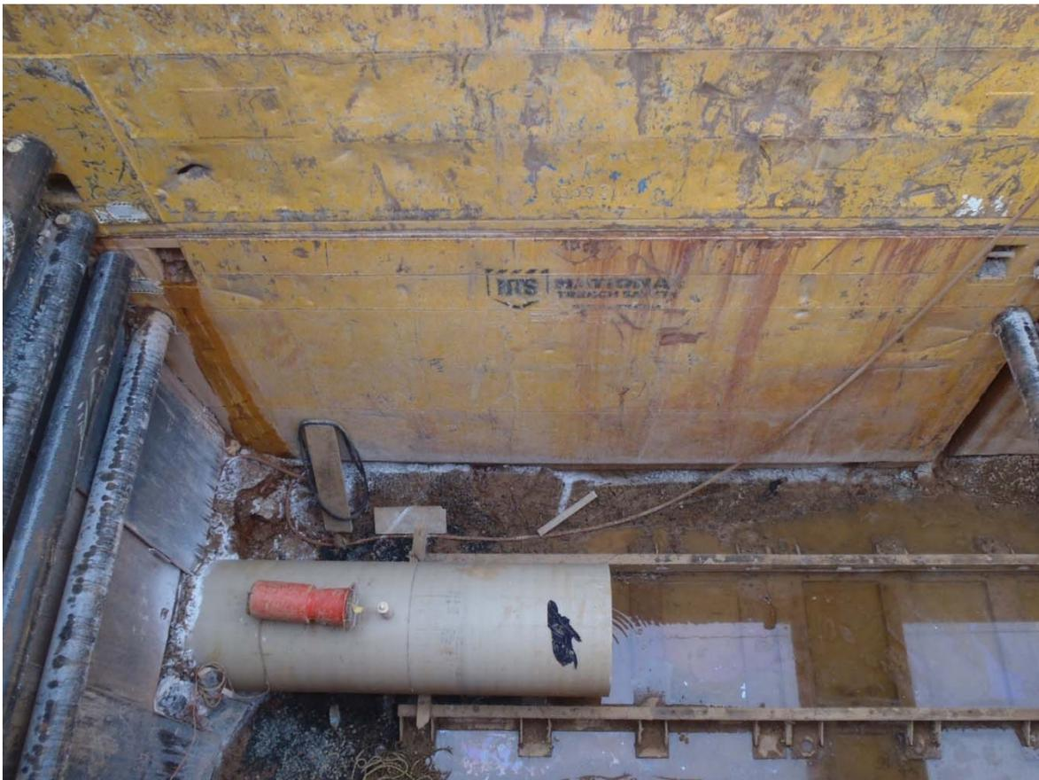
Figure 8 - Pipe Jacking Shaft
