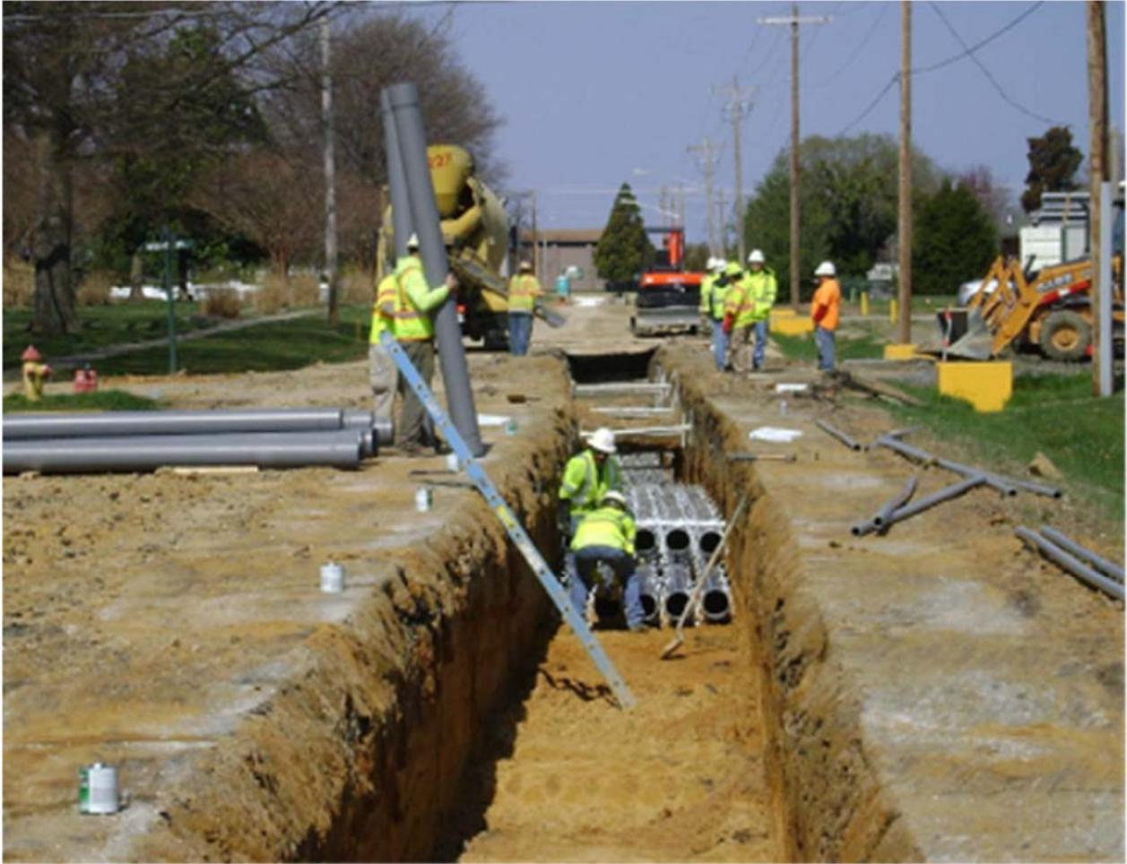
*Figure 1 - Duct Bank Excavation*
