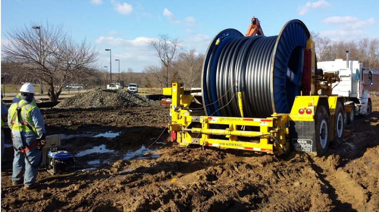
Figure 11 - Cable Reel Trailer
