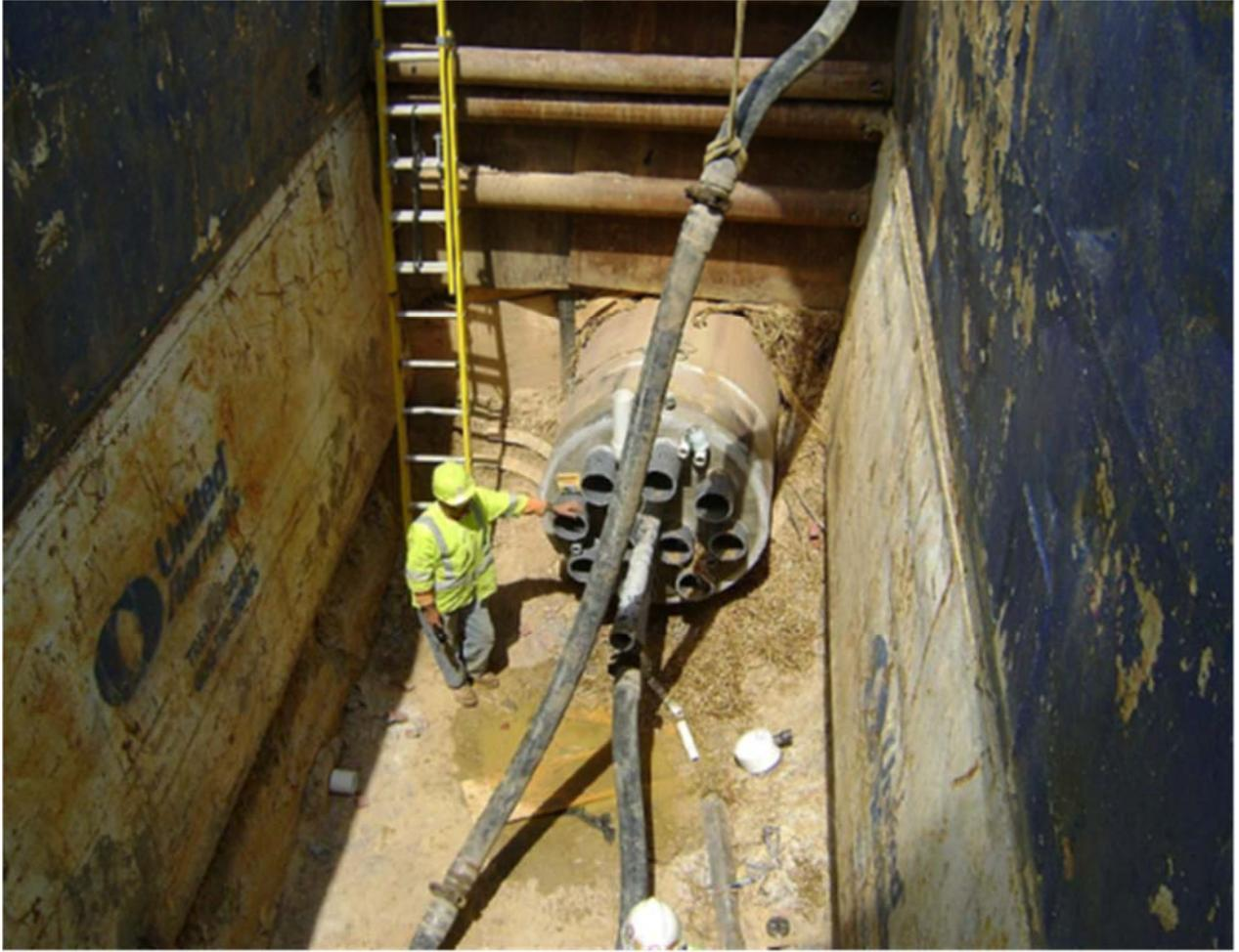
*Figure 9- Pipe-Jacking Shaft*
